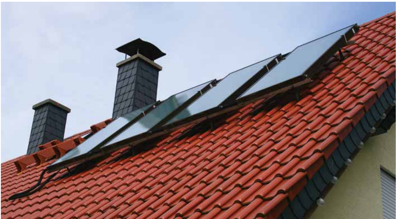
In solar panels, a solution of DOWCAL™ 200 fluid absorbs solar heat, and transports the energy so it can be used to heat water or air.
